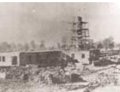
Crematorium II in its very early stages of construction.
